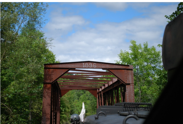
Photo 2: CCV Bridge with the year built punched in the steel.
