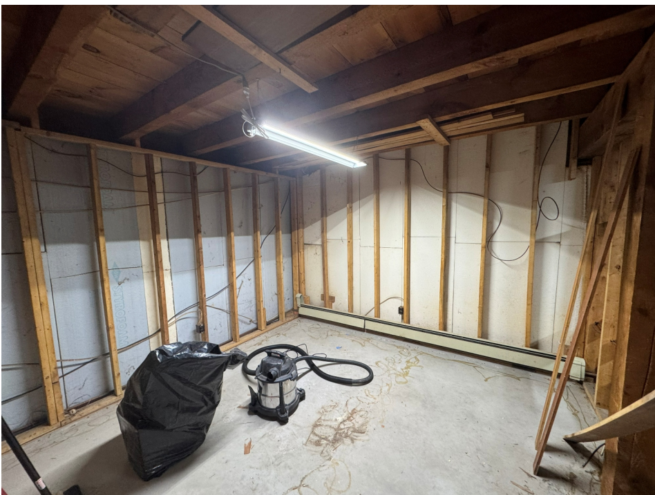
The layout room as viewed from the doorway into the room.
